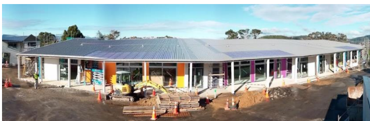
Photo of our new building
